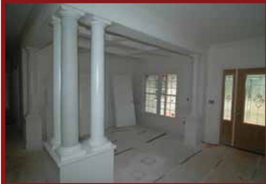
Coffered Ceiling & Columns in Dining
